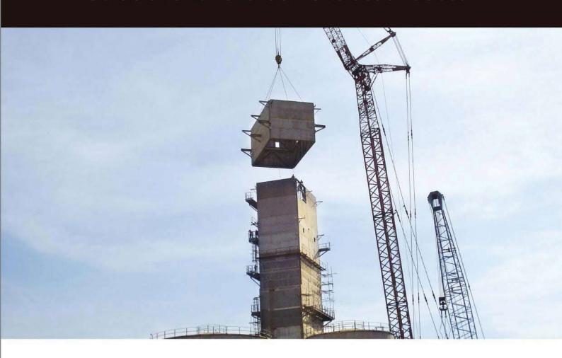
The project comprised placement of a 55 ton cold box at a height of 25 meters from the ground, at a radius of 22 meters with a boom length of approximately 63 meters. The movement and placement of the crane in a running plant was a challenge due to shortage of space, which was overcome with minor dismantling and skills of the operating crew.
